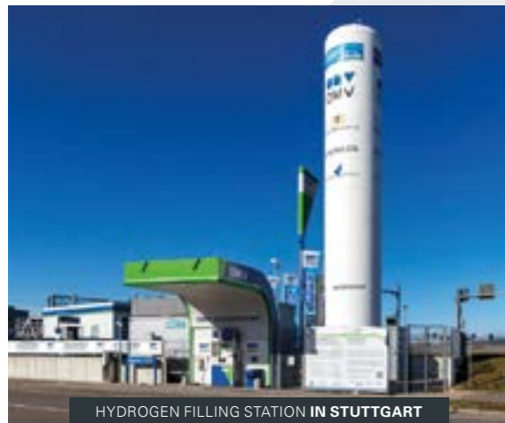
HYDROGEN FILLING STATION IN STUTT GART
